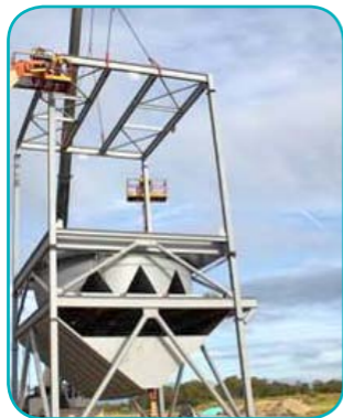
Partially completed assembly of QER's retort feed test unit (RFTU).
